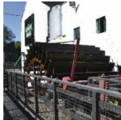
The waterwheel restoration project in Kilbeggan Distillery, Kilbeggan, Co. Westmeath used European larch sourced in Coillte forests in Co. Tipperary and sawn by Patrick Sheehan Sawmills Ltd., Clogheen. The project won a merit award in Wood Awards Ireland 2014, organised by the Wood Marketing Federation.
